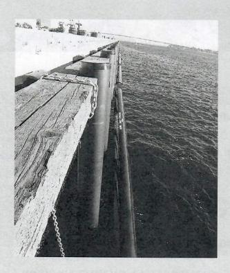
A variety of composite materials are available for their construction. The use of these materials provide a high strength positive buoyancy camel.
